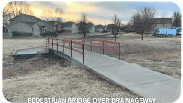
PEDESTRIAN BRIDGE OVER DRAINAGEWAY
