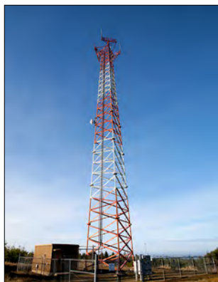
SELF-SUPPORTED LATTICE TOWER
