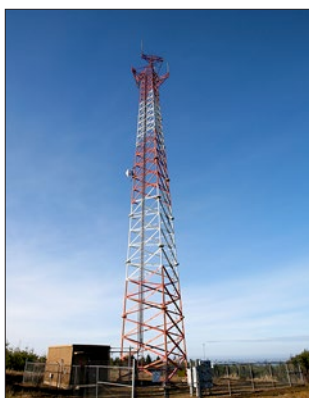
SELF-SUPPORTED LATTICE TOWER
